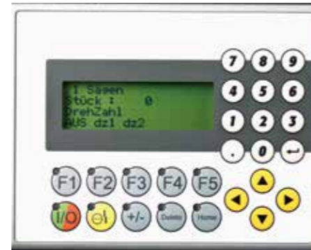
Input and diagnostic panel for operating and programming.
